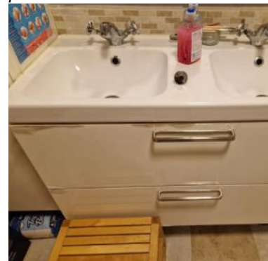
Water damage on sink unit from frequent use
